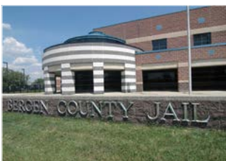
Bergen County Jail 820 MOBOTIX Cameras, U.S.A.
