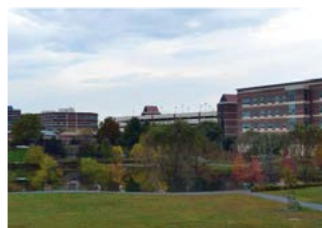
Valley Health Hospital 100+ MOBOTIX Cameras, U.S.A.
